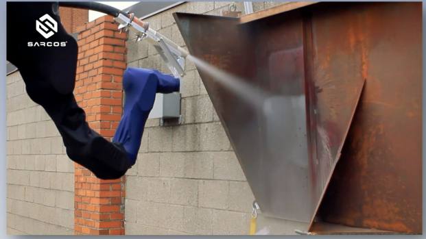
Media blasting to remove paint & rust
